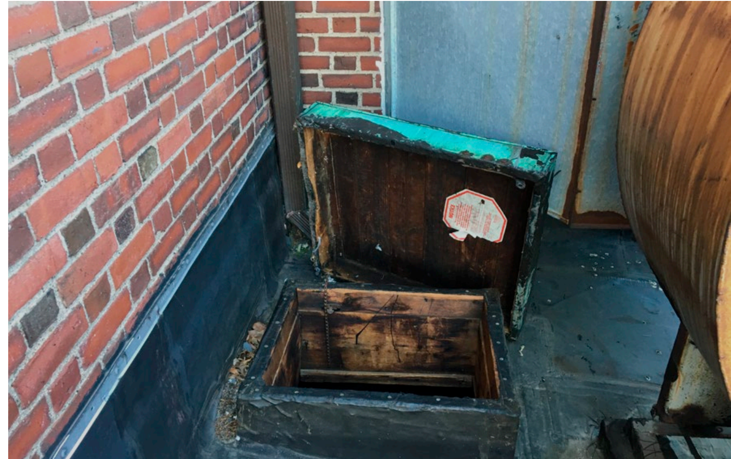
NON-SECURE ROOF ACCESS HATCH
