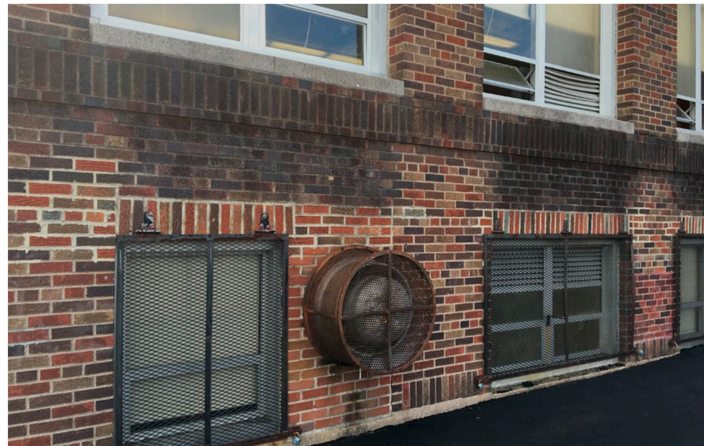
EXISTING WINDOWS ARE SINGLE PANE AND INEFFICIENT
