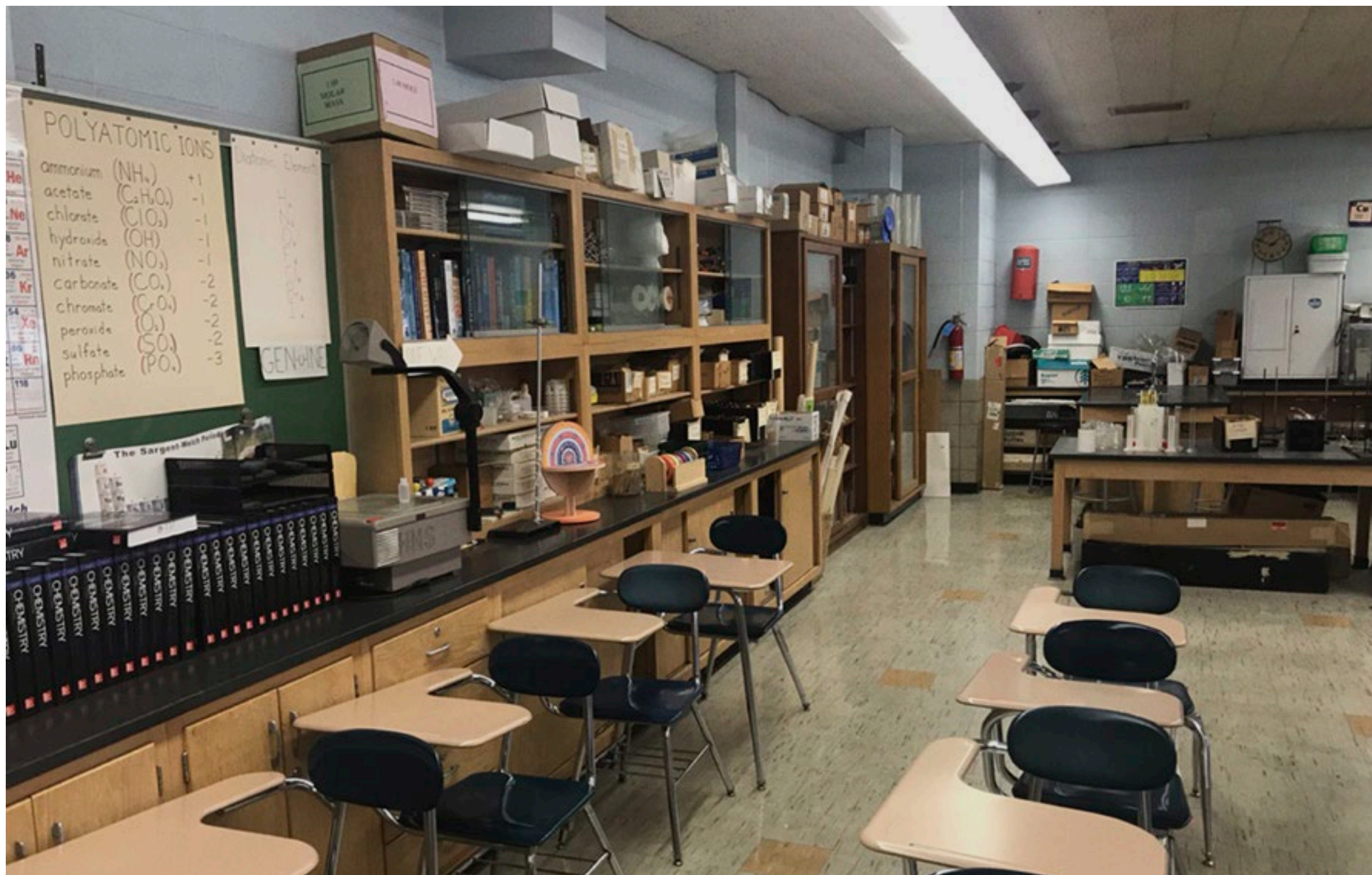
SCIENCE LABS WITH ORIGINAL CASEWORK, COUNTERTOPS AND WORN 9X9 FLOOR TILES
