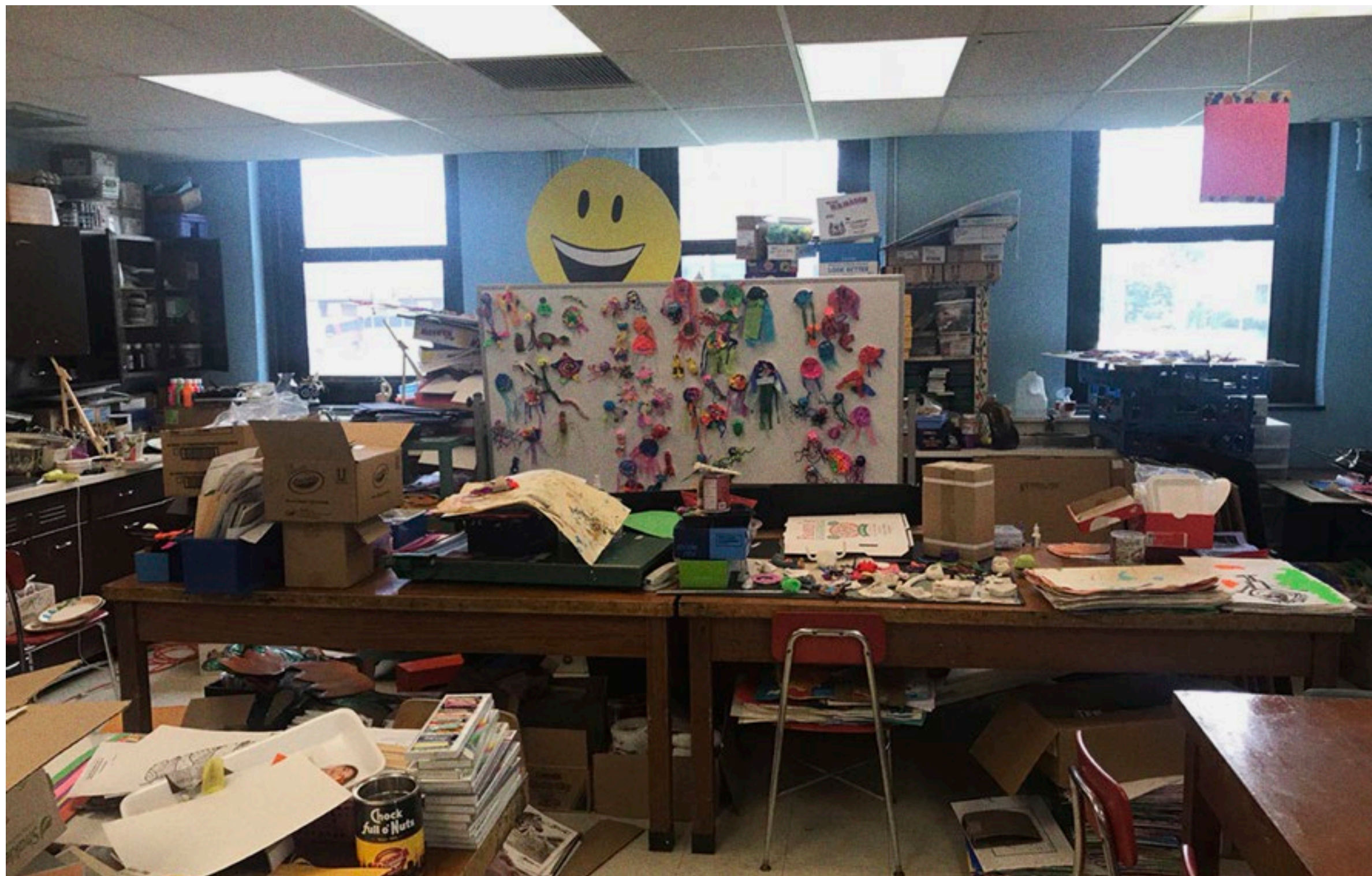
ART CLASSROOM – DATED, OLDER, INSUFFICIENT POOR STORAGE; DIFFICULT TO SUPPORT GROWING CURRICULUM
