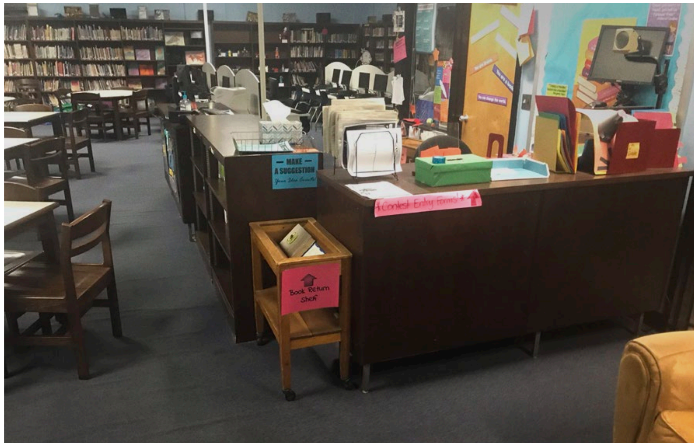
EXISTING LIBRARY - OLDER, INEFFICIENT, UNABLE TO SUPPORT EVOLVING CURRICULUM; LOOSE CARPET PRESENTING TRIPPING HAZARD
