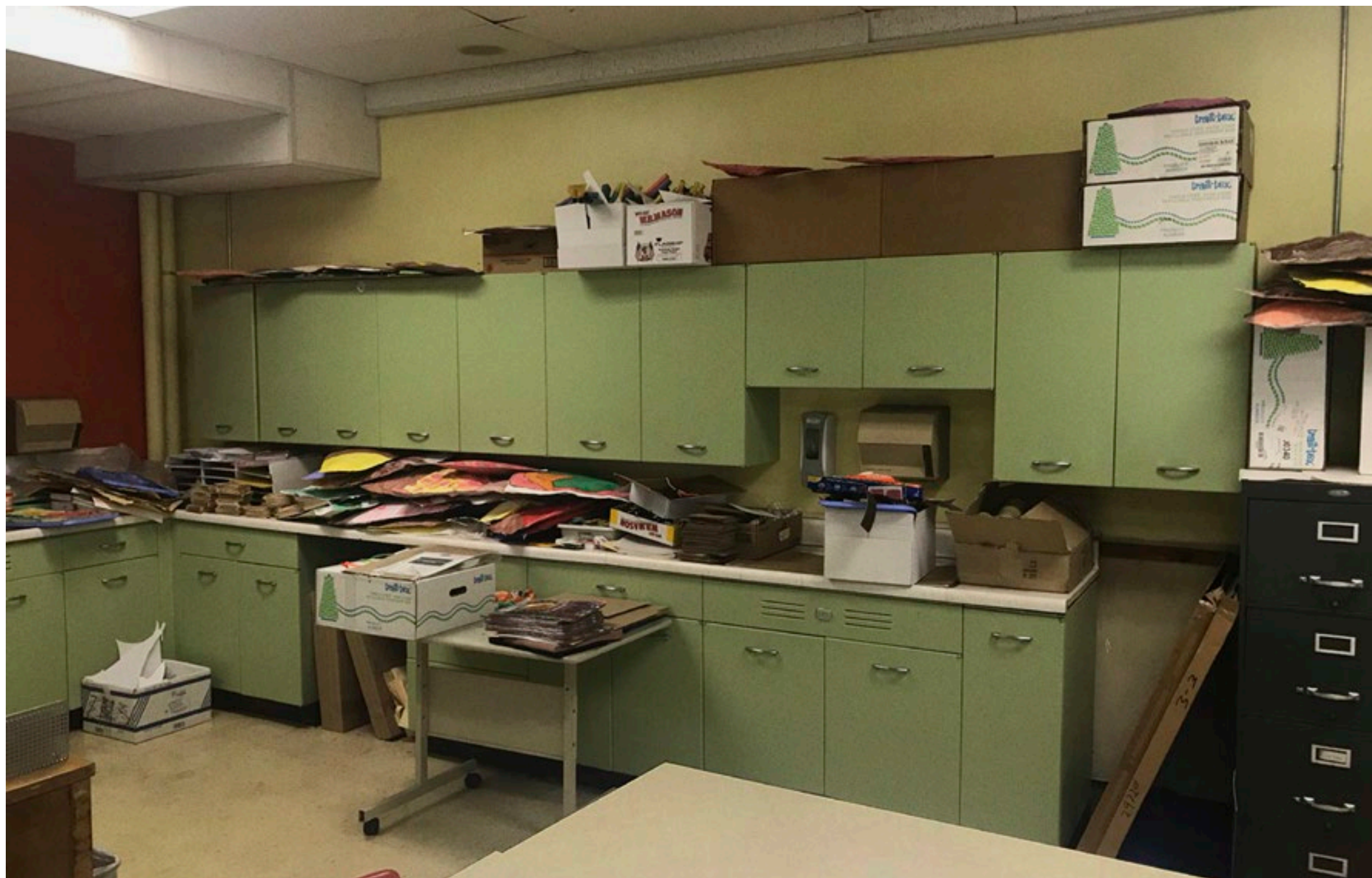
ART CLASSROOM – DATED, OLDER, INEFFICIENT STORAGE; DIFFICULT TO SUPPORT GROWING CURRICULUM
